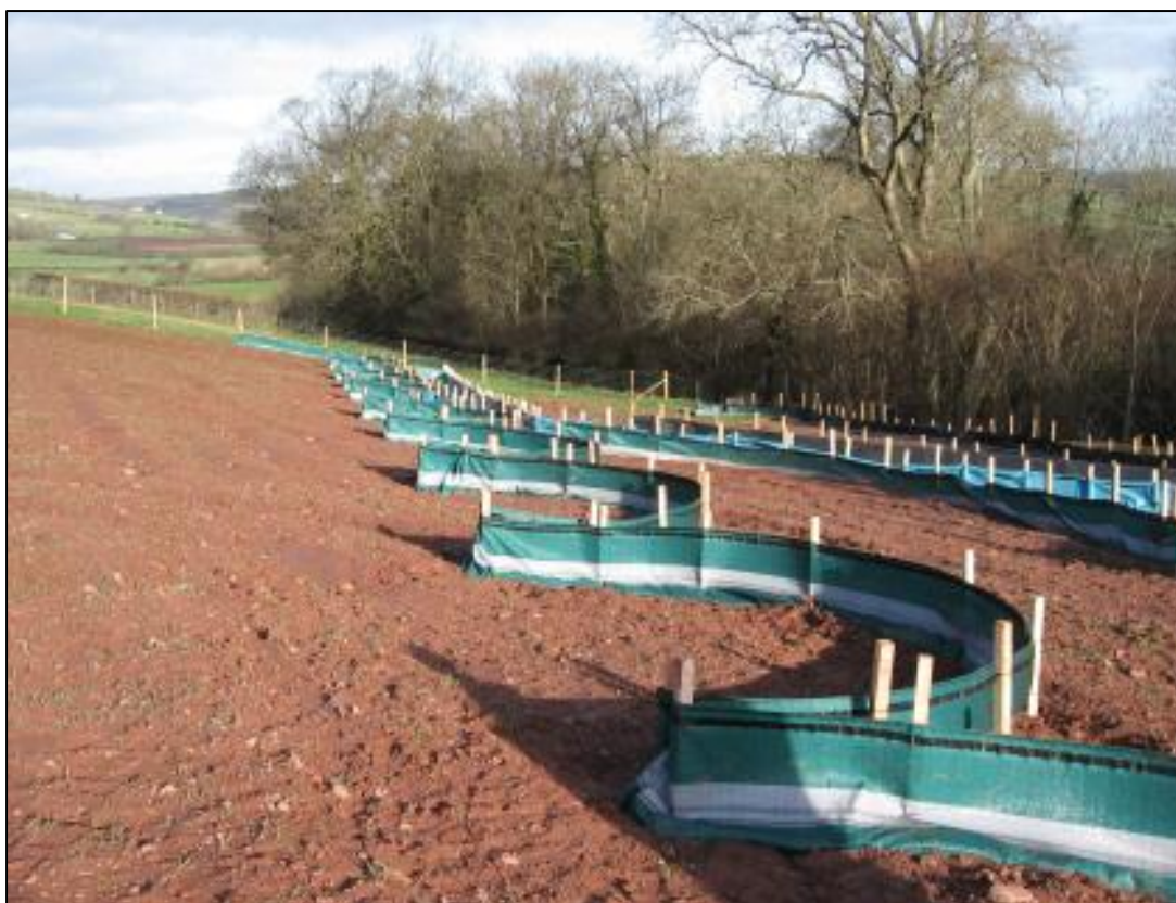
Plate 2 – Example of good practice in silt fence installation (Source: Geosynthetics, 2021 11 )
